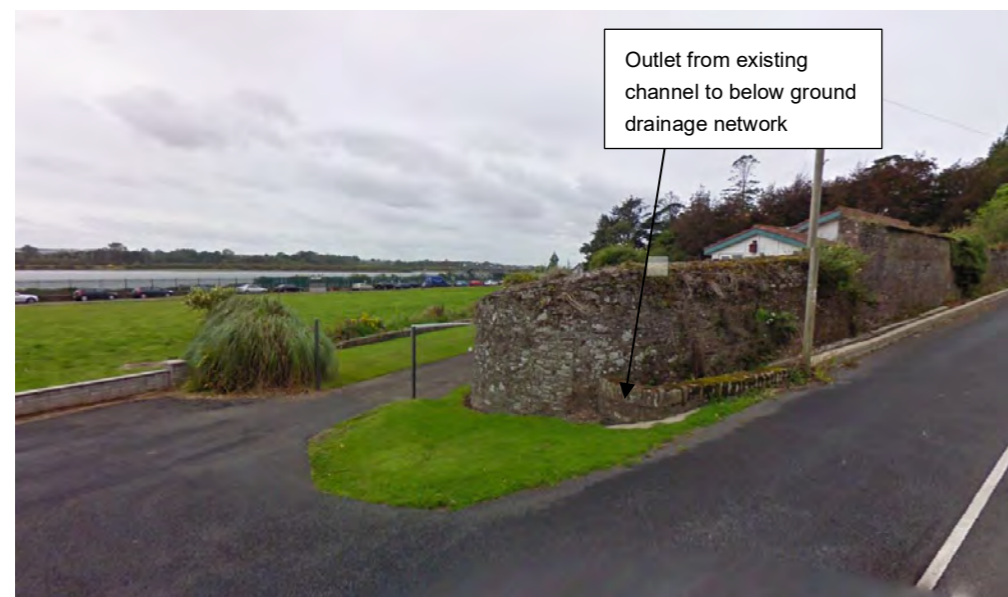
Figure 2-2 – Existing Channel on the Terrace/ Johnstown Close
