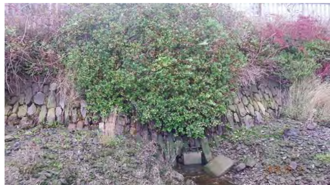
Figure 2-3 – Existing Outfall at Glounthaune Train Station
